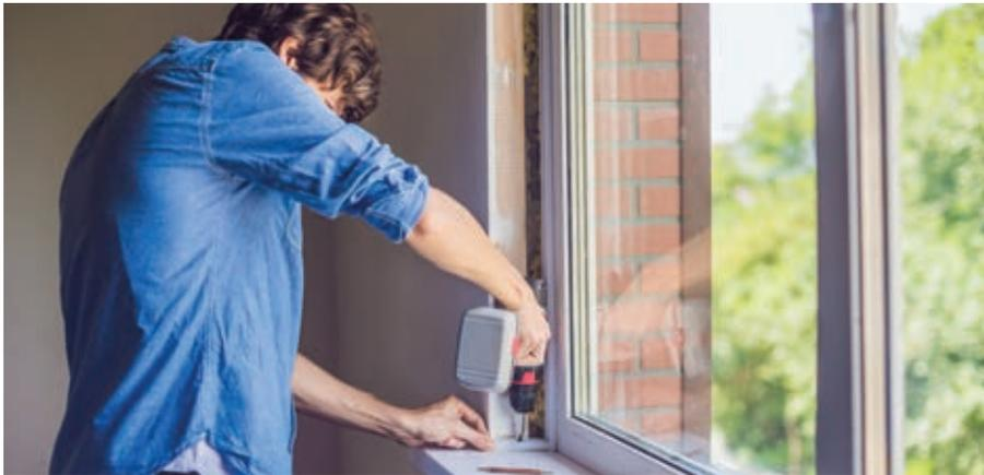
The seam between the window frame and the wall is a common source of air leakage. Fill gaps less than 1/4-inch wide with caulk; for larger gaps, use expanding foam and paint over it.
